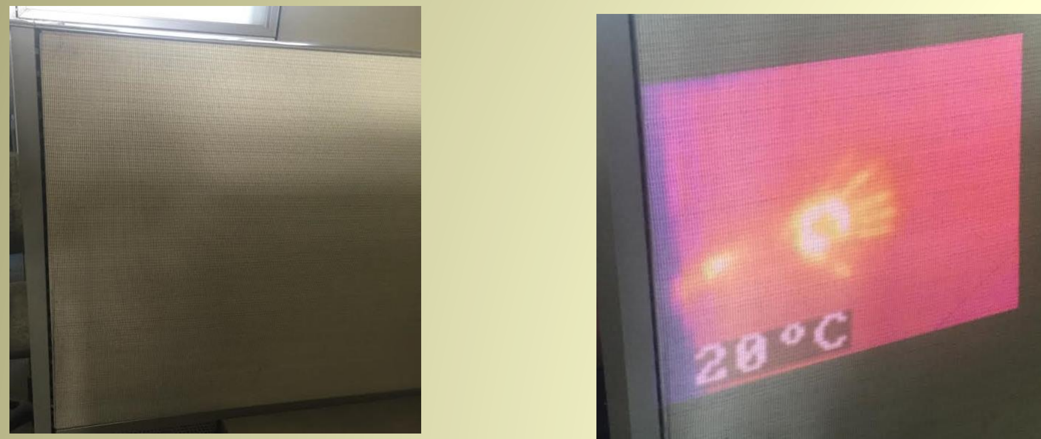
Figure 1. What the naked eye sees (left), the thermal gradient revealed by the Flashlight (right)
