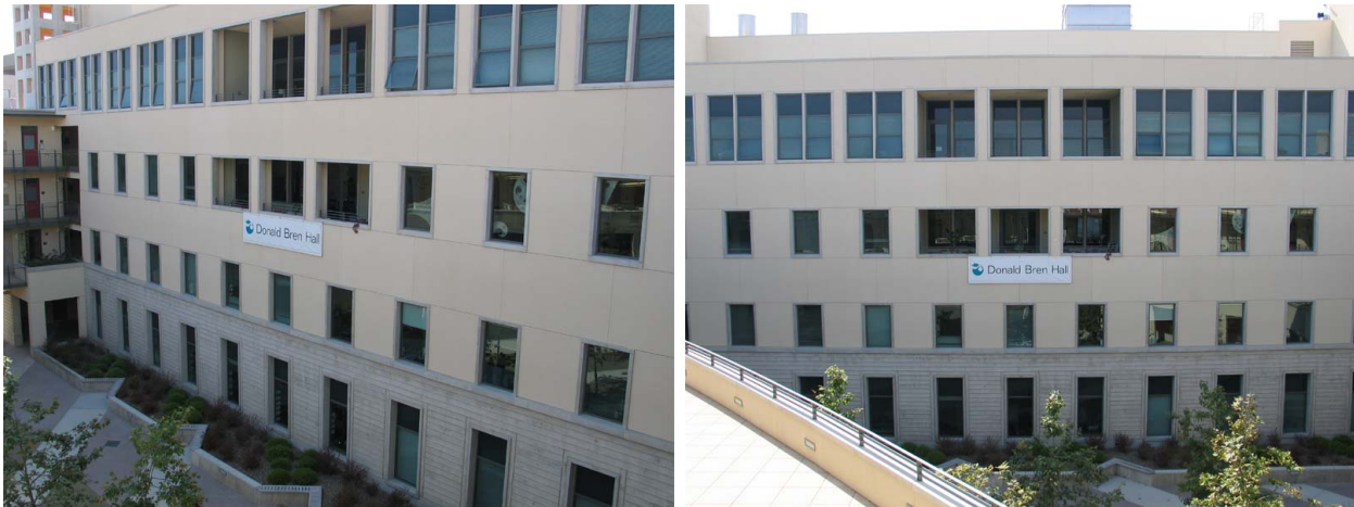
Fig. 1. The left images shows one of the almost planar facades of the Bren School with a large perspective distortion. The goal is to construct a projective transformation that rectifies the image producing a result similar to the right image.
